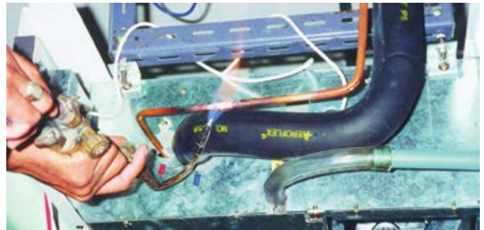
Self-extinguished property, low smoke density, less toxic gases and non-melting characteristic when burnt, making Aeroflex widely used in air-conditioning systems.
